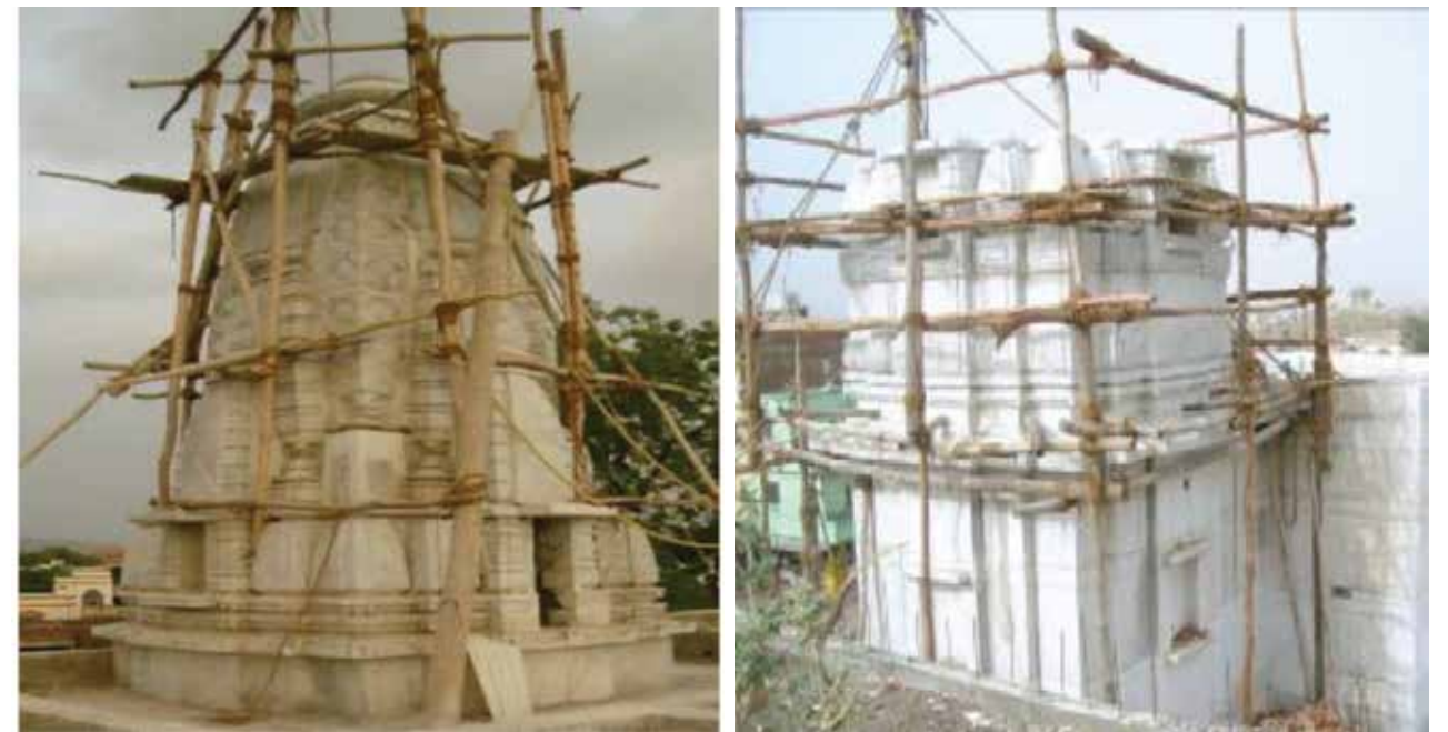
fig.23 The process of construction of sikhara
