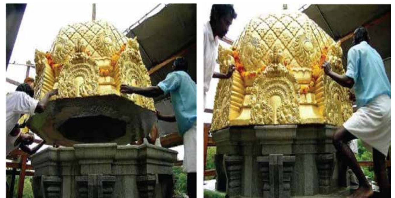
fig.25 The process of placing the cap stone or sikhara
