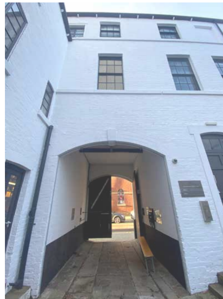
Cart entrance from the courtyard
